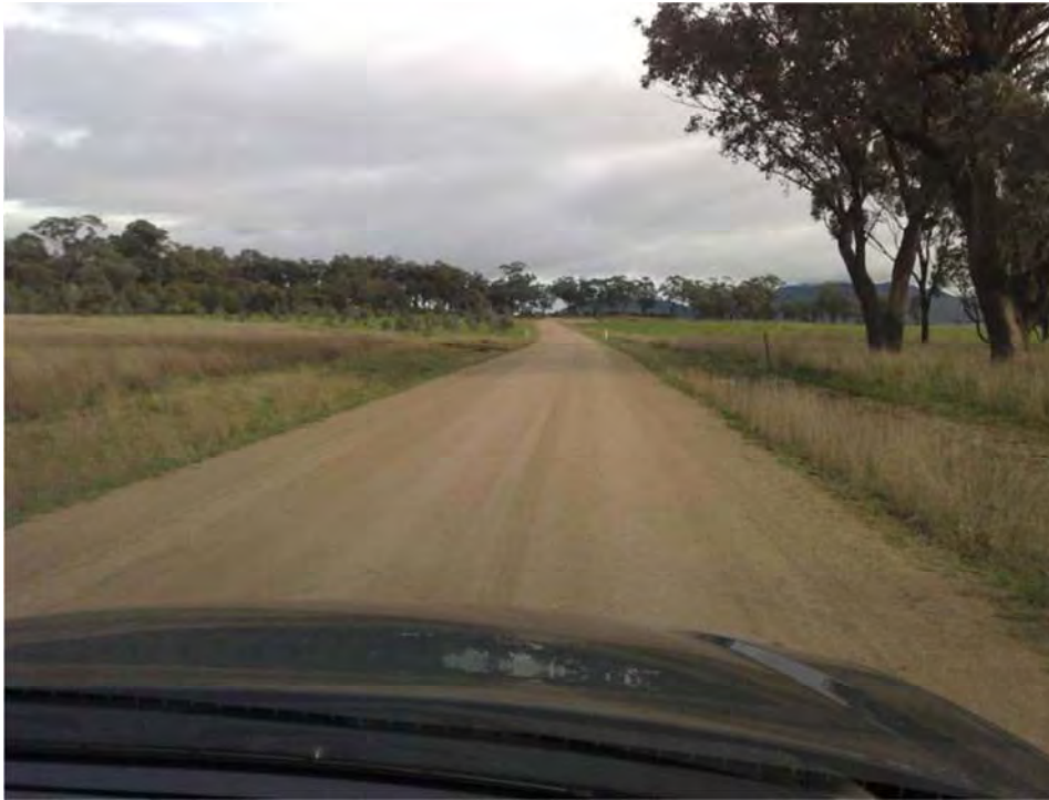
Plate 1 Escott Road Typical Alignment and Condition
