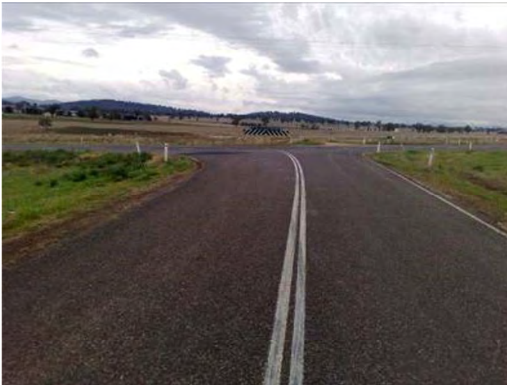
Plate 9 Taylor's Lane Intersection with Werris Creek Road
