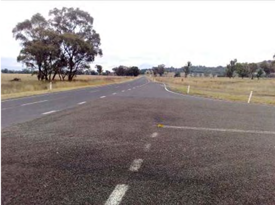
Plate 12 Taylor's Lane Intersection Looking Towards Gunnedah
