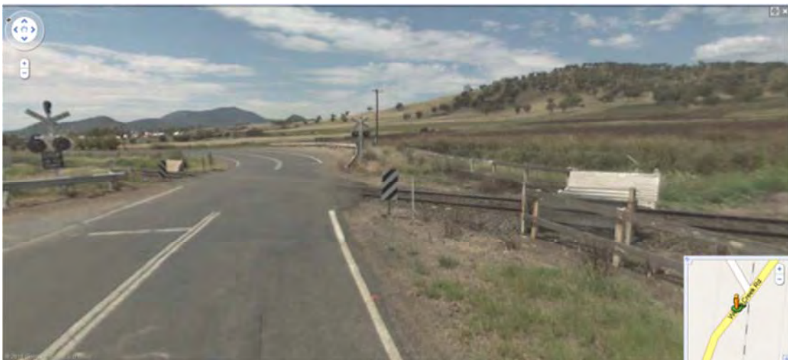
Plate 21 Level Crossing at Werris Creek Road South Werris Creek
