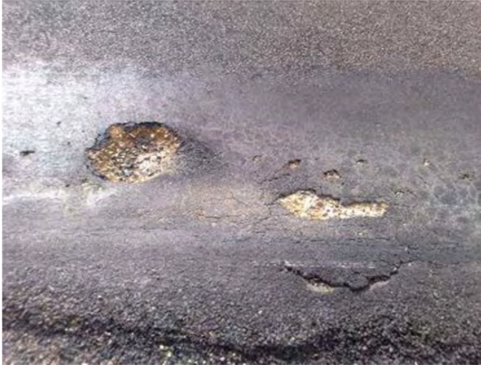
Plate 4 Taylor's Lane Pavement Failure
