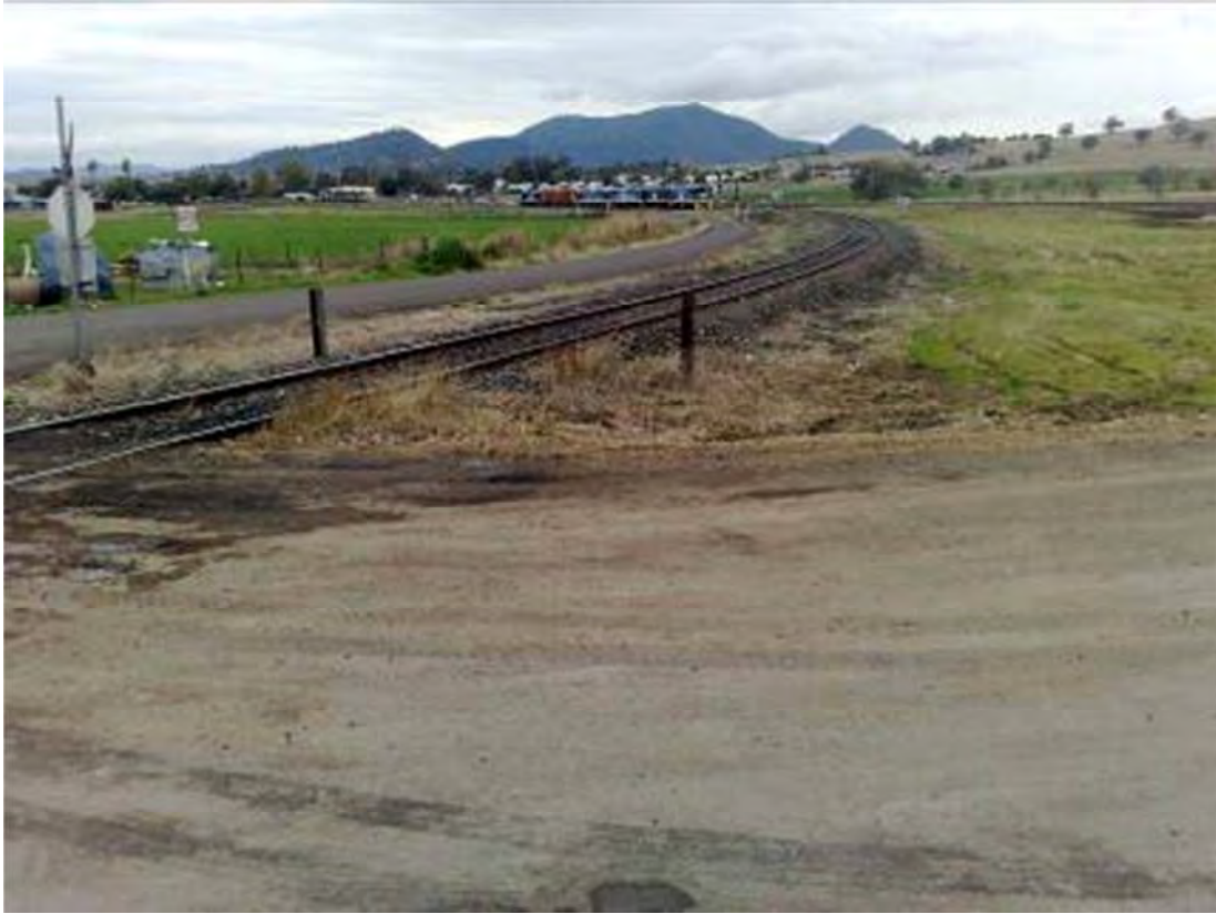
Plate 20 South Street Crossing Looking Along the Maintenance Facility Access
