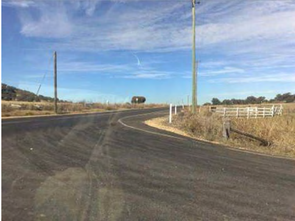
Plate 8 Escott Road Intersection Looking South Towards Quirindi
