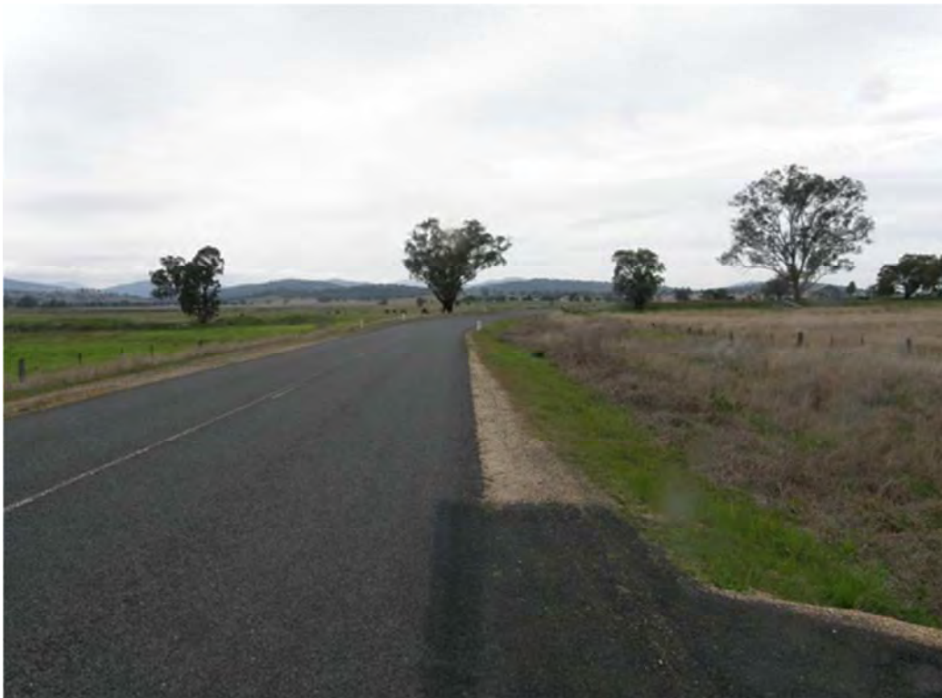
Plate 5 Taylor's Lane Driveway Access Close to Bend (Approximately 575m from Werris Creek Road Intersection)
