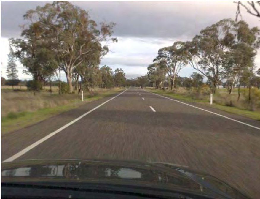
Plate 6 Kamilaroi Highway Typical Alignment and Condition
