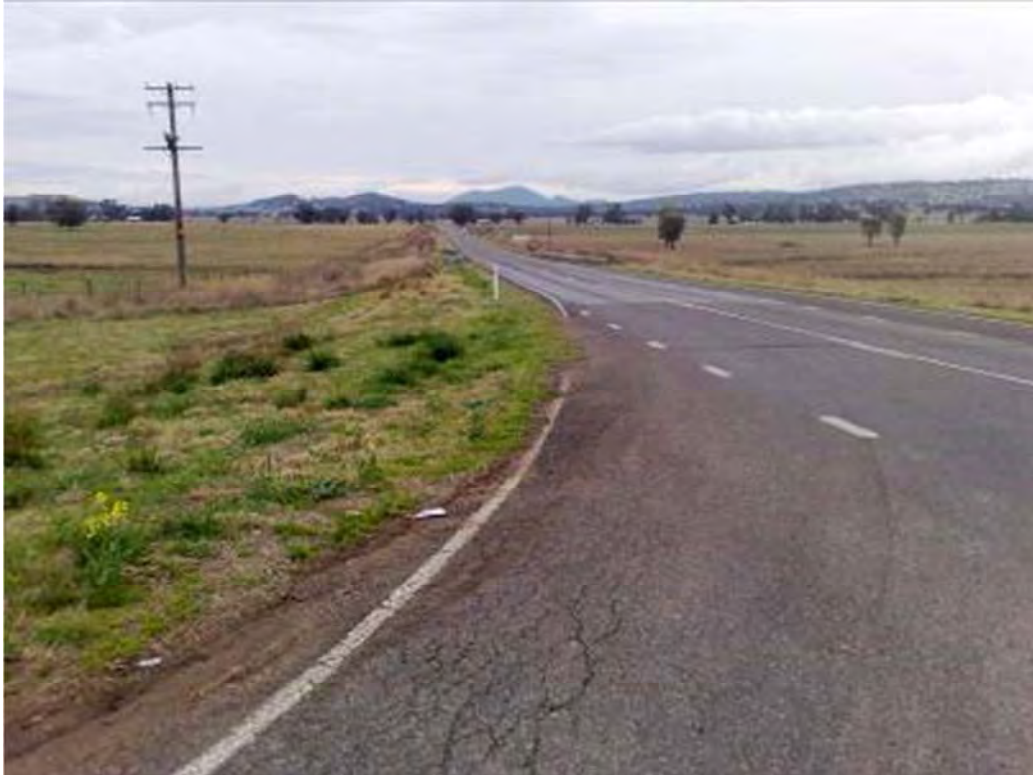
Plate 11 Taylor's Lane Intersection Looking Towards Werris Creek
